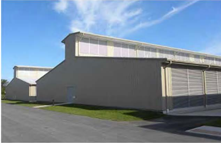
Yahoo Server Farm, intake along the bottom, outflow at top.
